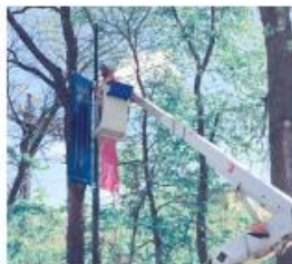
Installing Decorative Banners
